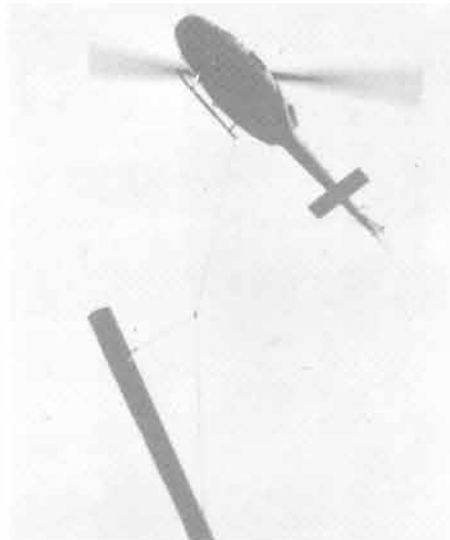
Bell 212 transferring building materials to Catherine's Peak.
